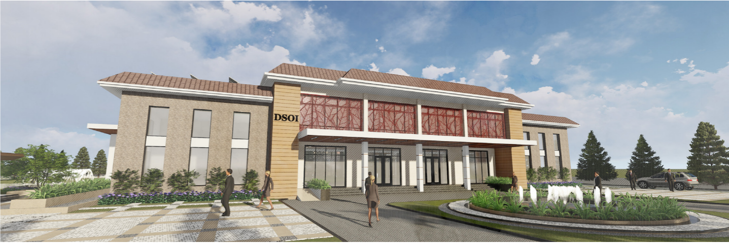
Maximum exposure North-south. Grass concrete pavers on peripheral roads to extend visual size of banquet lawns . Due to the building placement north-south, maximum shade in lawn and courtyards.
